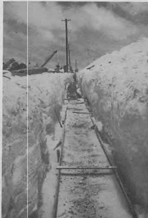
POWER DISTRIBUTION ducts and cables went underground to replace the vulnerable overhead system.
