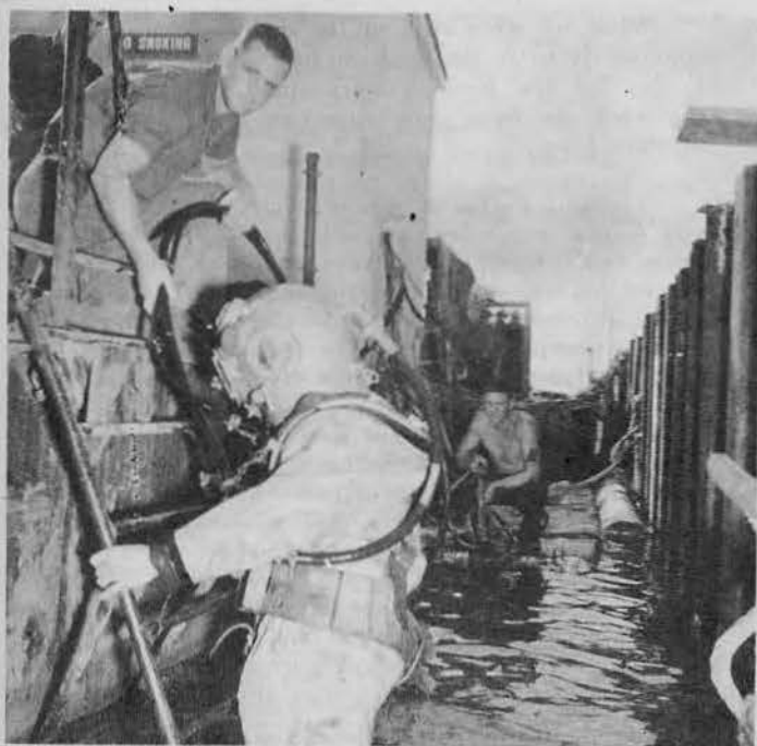
BATTALION DIVERS often braved swift currents and sharks in carrying on the very necessary underwater construction and salvage work. In the picture Tom Kallison (in suit) is tended by Harry Heinemann and Fred Hall.
