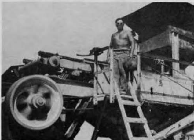
JENKINS and his crusher processing the coral for runway surfacing.
