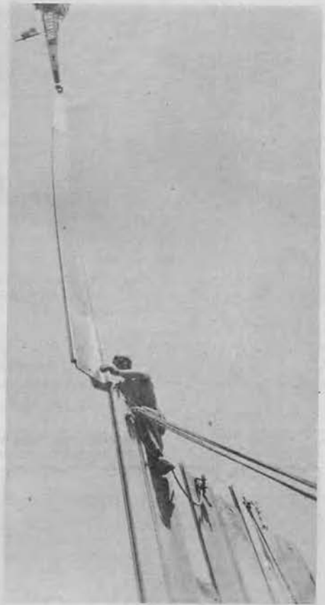
Sheet piling being guided into slot by agile rigger.
