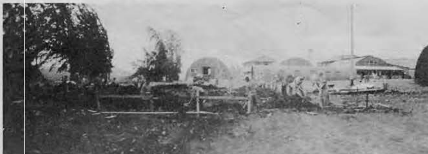
"SHOVEL OPERATORS" excavating for a Ship's Service store built by the Battalion on Oahu.
