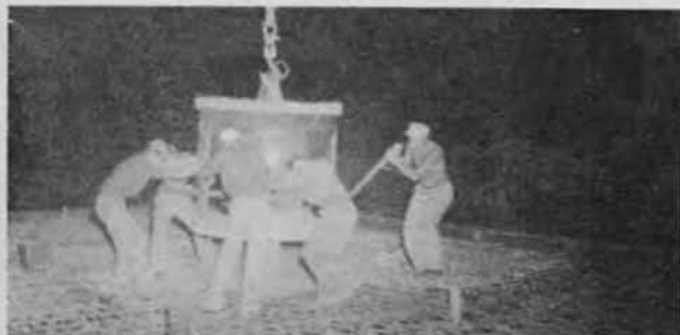
CONCRETE being placed at night in a large continuous pour.
