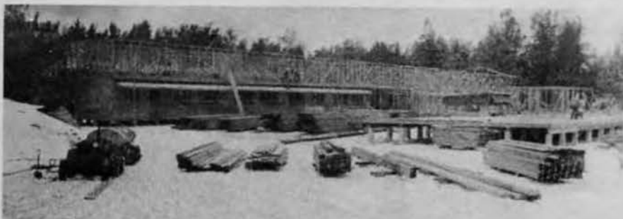
FRAMING going up for a two hundred man BOQ on "Island X."
