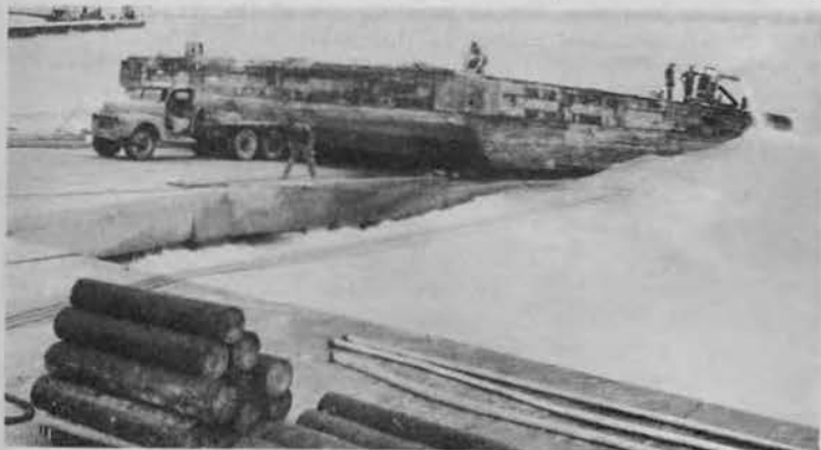
BEACHING a 150 ton barge required some ingenuity, rigging and equipment.
