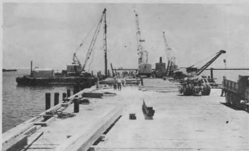
FENDER PILING being driven while decking continues on this large pier.
