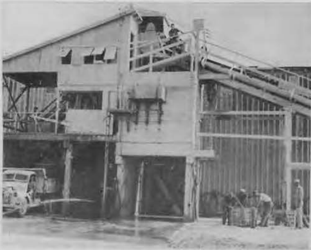
Truck backing under concrete mixer during a large continuous pour.
