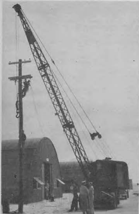
HIGH WIRE ARTISTS performing in the act of getting a transformer into place.
