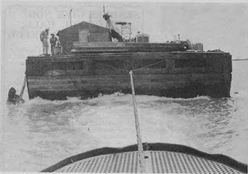
The pile driving barge, although big, was easily towed between jobs by Stout's tug "Jerry."
